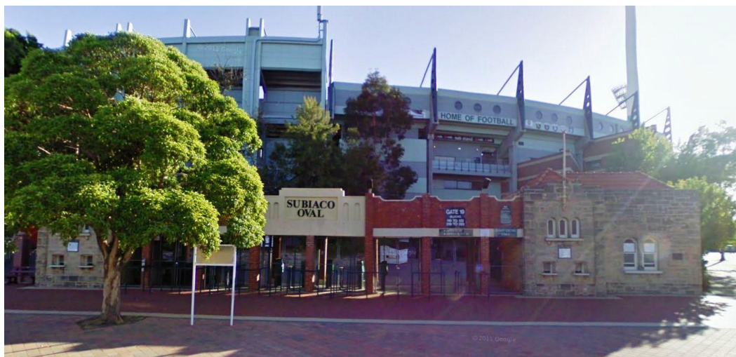
Entrance gates at Subiaco Oval designed by Alfred Wright in 1935 - a familiar sight to many Western Australians (Google 2013).
